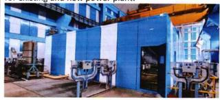
Silencers are provided to high pressure steam vents (as per photograph below) to control noise.
